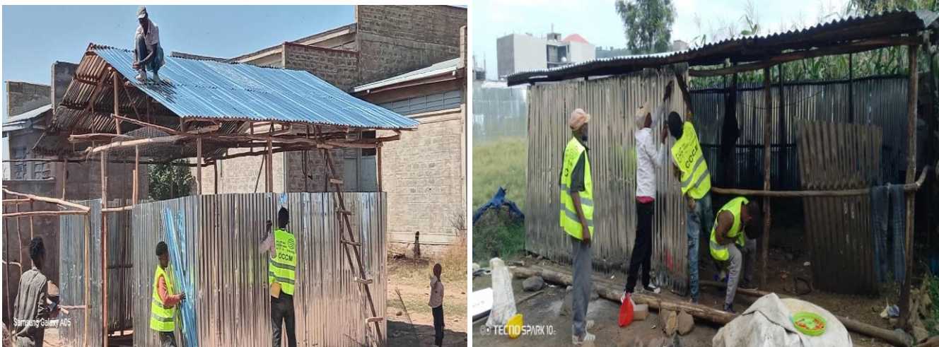
Construction of a communal kitchen to support shared cooking and improve living conditions.
