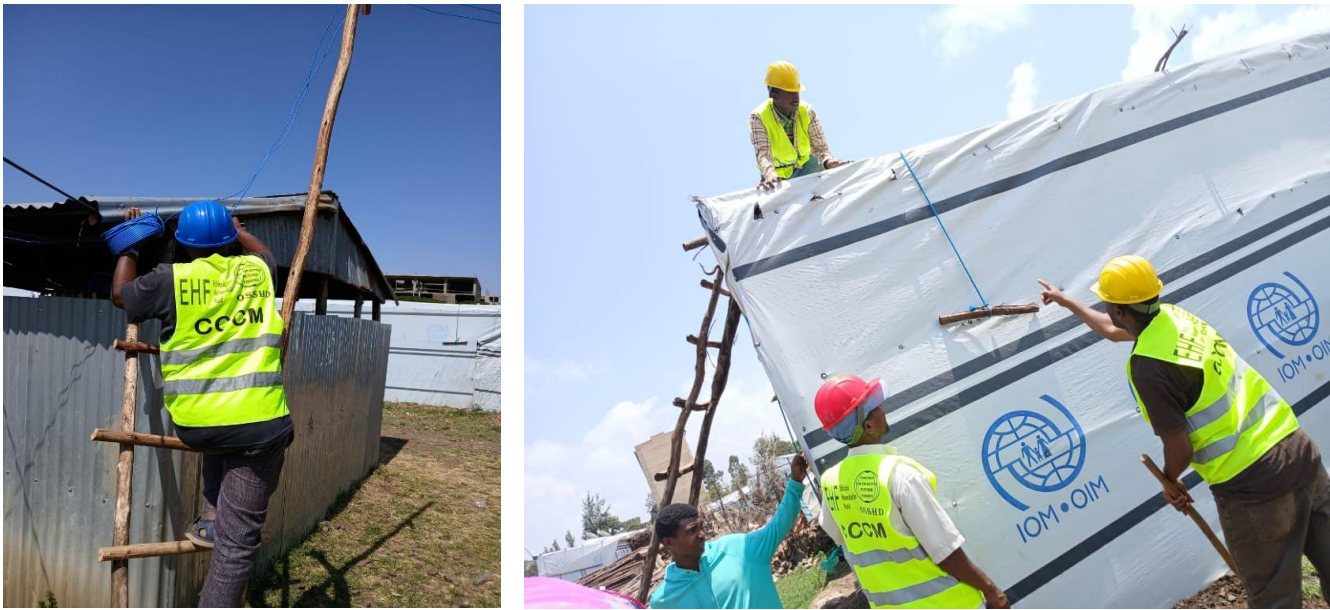
Shelter maintenance committee actively engaged in on-site shelter repair activities.
